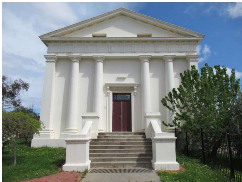
February 2023. Eaglehawk East Uniting Church – Former. Source: Australia's Christian Heritage, churchesaustralia.org .
