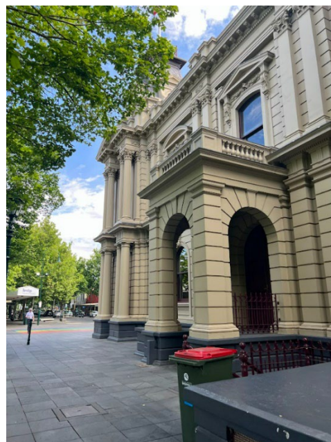
2023. Entry portico, western façade near Hargreaves Street.
