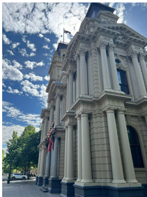
2023. Detail of façade columns.
