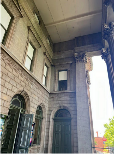
2023. Inside entrance portico, view of Corinthian column.
