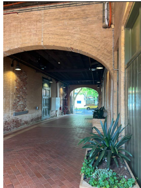
2023. Ground level right of way to ground floor of 1890 extension.
