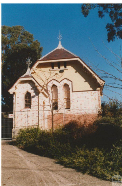
Little Bendigo Primary School, 2010. This picture was taken during restoration works, when non-original paint (seen in the top section of the building) was removed to restore the original red brick. Photographer: John Young. Source: Victorian Places ( victorianplaces.com.au )
