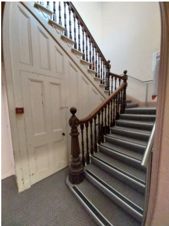
2023 timber joinery to internal staircase.
