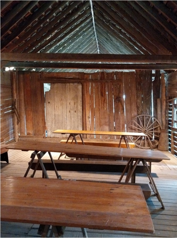
2023. Shingle ceiling in the Shed.
