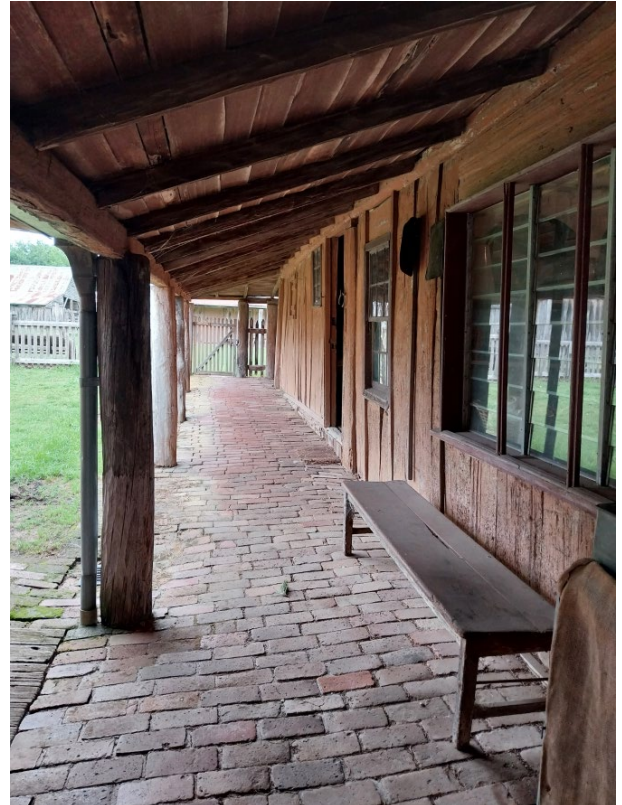
2023. Verandah to kitchen block.
