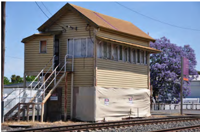
2024, north and east elevations of Benalla Railway Signal Box with external stair accessing the operating room and external toilet. Source: Heritage Victoria
