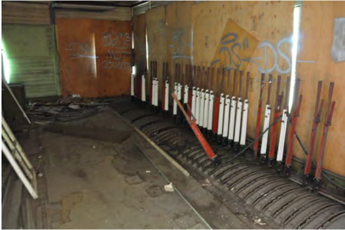
2024, interior of operating room (upper level) with signal and points levers set in McKenzie and Holland lever frame. Source: Heritage Victoria
