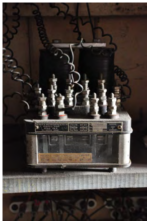
2024, signal relay located in locking room. Source: Heritage Victoria
