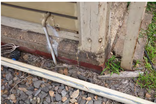
2024, detail of corner post supported on a brick and concrete base, with aluminium cladding, Source: Heritage Victoria
