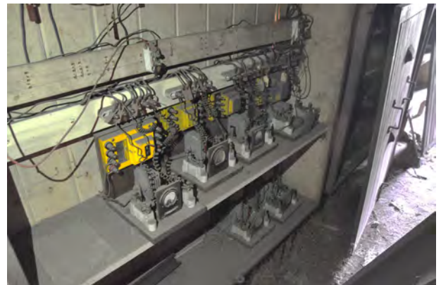
2024, electricity transformers and ammeters located in locking room. Source: Heritage Victoria
