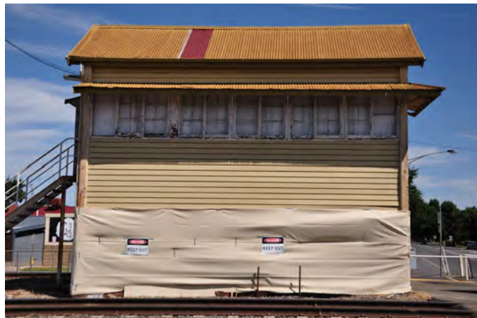
2024, north elevation of Benalla Railway Signal Box with temporary fabric covering to locking room following a vehicle strike. Source: Heritage Victoria
