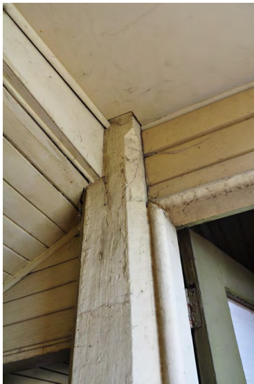
2024, detail of chamfered corner timber post. Source: Heritage Victoria
