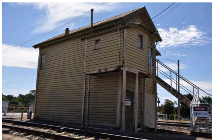
2024, south elevation of Benalla Railway Signal Box featuring external stair accessing the operating room and external toilet. Source: Heritage Victoria
