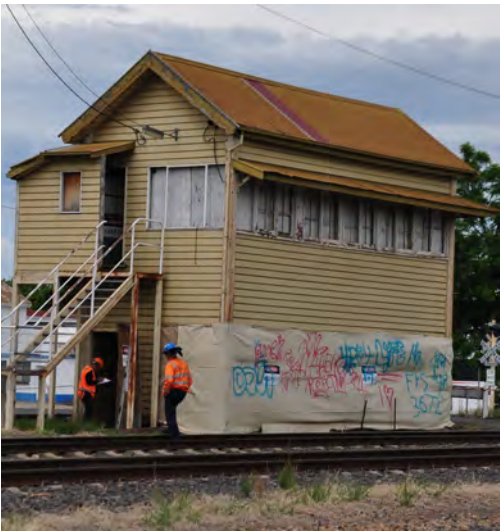
2024, fabric covering the exterior to the locking room (ground floor) following vehicle strike
