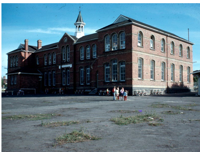
Gold Street Primary School, photographed around 1970 by Laurie Burchell. From Laurie Burchell collection, State Library of Victoria. This shows the southern elevation of the building, which has now been renovated and is largely obscured by a modern construction.
