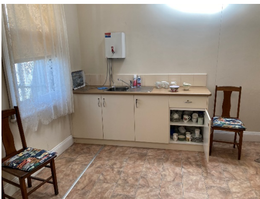
2022, Warracknabeal Ladies Rest Rooms, kitchen sink area
