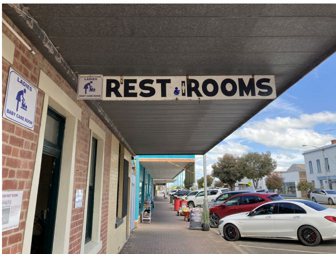
2022, Warracknabeal Ladies Rest Rooms, view south along Scott Street
