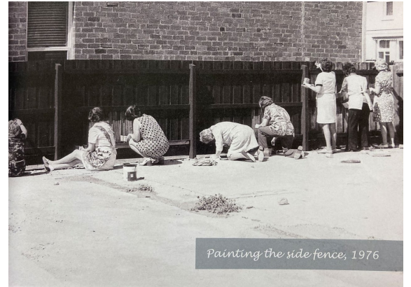
1976, Painting the side fence, Source: Graeme Massey, Warracknabeal Ladies Rest Rooms
