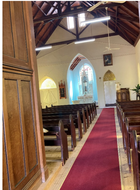
April 2023, Interior view from the south to the north of the church
