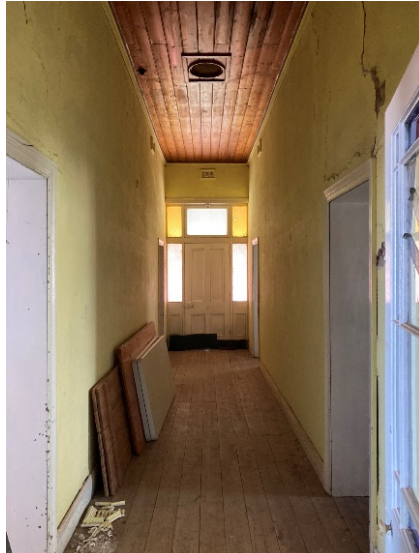
April 2023, Interior corridor looking north to south
