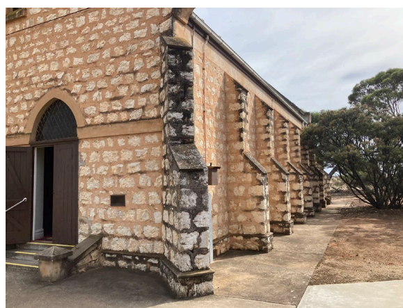
April, 2023, Southeast elevation of church
