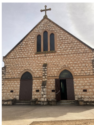
April, 2023, Southern elevation of church (front entrance)
