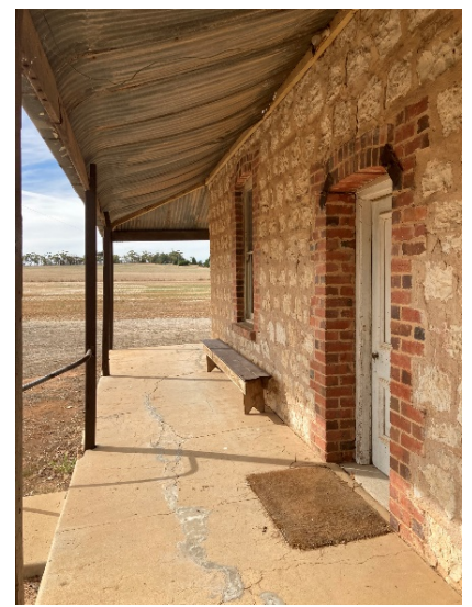
April 2023, North verandah looking east
