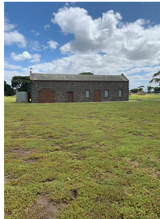
View of stable building. (Image: Parks Victoria)
