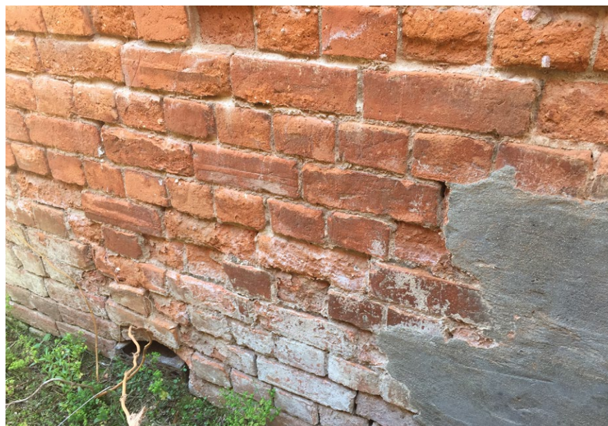
Drainage issues at the base of the building will result in movement in the shallow stone footings and consequent cracking of the walls.
