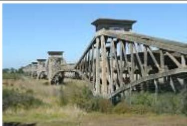
The **Ovoid Sewer Aqueduct** over Barwon River, Geelong (VHR H0895), is significant as an outstanding application of the Considere system of concrete reinforcement in a design derived from the steel Firth of Forth Bridge in Scotland. It enabled an overall length and span which exceeded any other reinforced concrete structure at the time of construction.
