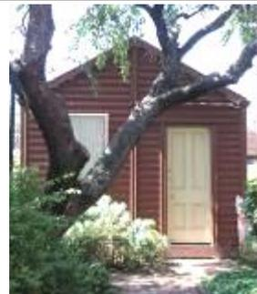
The **Bellhouse Iron House**, South Melbourne (VHR H1888), is significant as one of the few surviving examples of prefabricated, portable iron housing imported from England in the 1850s due to the rapid increase in population and scarcity of materials and labour during the gold rush.
