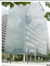
**ICI House**, Melbourne (VHR H0786), is significant for its considerable advancements in local construction techniques, including framed glazed curtain walls and innovative use of concrete, including precast reinforced units in structural members and flooring. The division of the glazed office space from the solidly clad service tower predates similar developments overseas.
