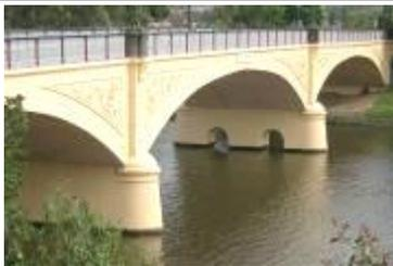
The **Morell Bridge** over the Yarra River at Anderson Street, South Yarra (VHR H1440), is significant as the first reinforced concrete bridge built in Victoria (1899) – only two years after the first reinforced concrete bridge in the world – and the first in Victoria to use the innovative Monier construction technique patented by Joseph Monier, a French manufacturer of garden ware.
