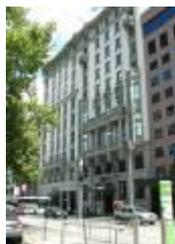
The **Commercial Travellers Association Building**, Melbourne (VHR H0934), is of architectural significance for a number of innovations, such as the use of welded wire reinforcing mesh, perhaps the first use of such material in Victoria, and 'Mack' slab cement partitions, the only known use of this technology in Victoria. It was also one of Australia's earliest steel framed buildings.
