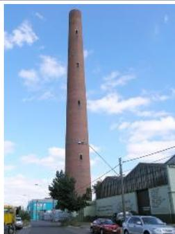
The **Shot Tower**, Clifton Hill (VHR H0709), is rare as one of two surviving shot towers in Victoria. Its form reflects the shot production process: the shot was produced by dropping molten lead through sieves at the top of the tower into water at the bottom. The height of the tower allowed the shot to form before reaching the bottom.
