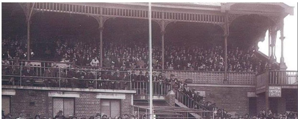
1933, Detail, Richmond's 1932 premiership flag is unfurled ... showing the low building installed in 1926-27 at bottom left. Source: Richmond FC website
