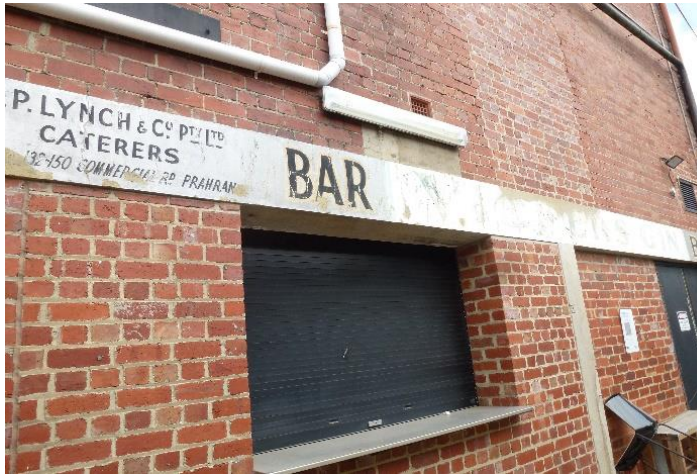
2022, Bar signage and servery window, Jack Dyer Stand
