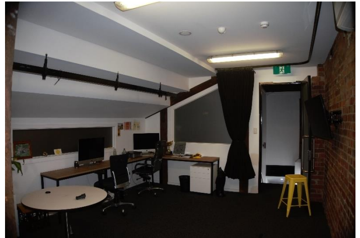
2022, Interior showing underside of tiered flooring of grandstand
