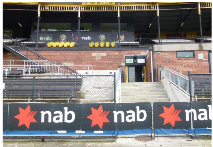
2022, New concrete tiered seating area
