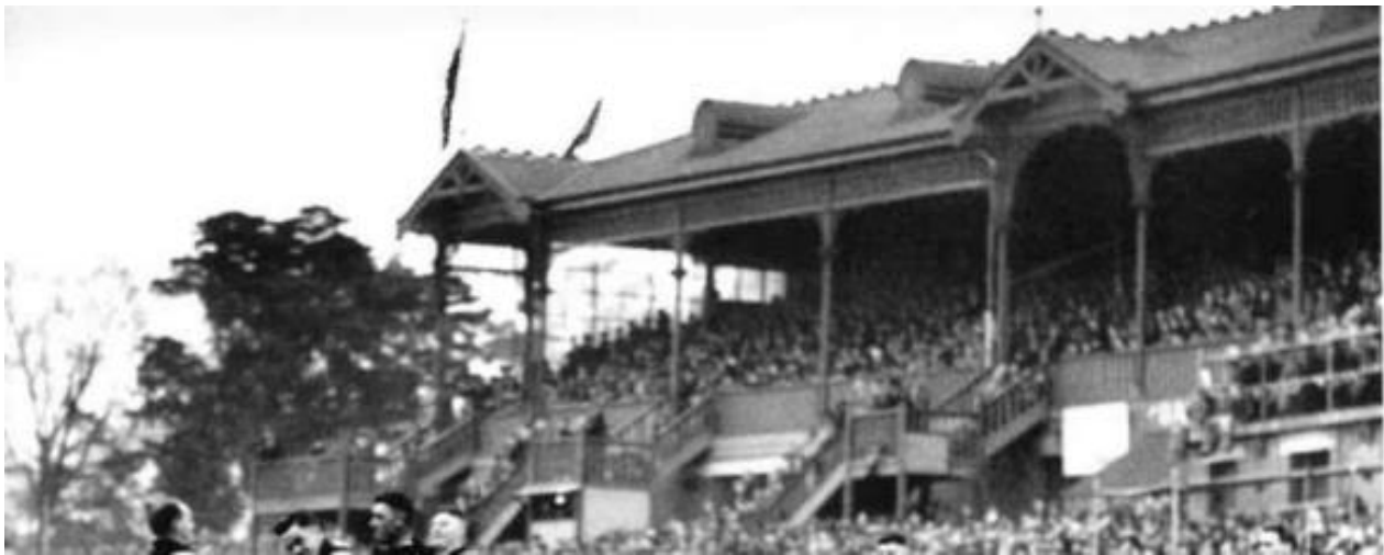
1927, Detail, new western extension to grandstand with three new staircases. The design continues the frieze, roof vents and ridging of the original grandstand. New low building with viewing platform roof to the right. Source: (Bartlett & Ruddell, 2012)
