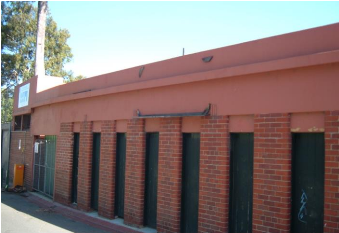
Undated, 1930s entrance gates, demolished ca. 2007. Source: The Holy Boots Football Emporium blog
