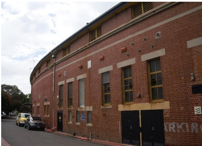
2022, Rear showing brickwork in good condition
