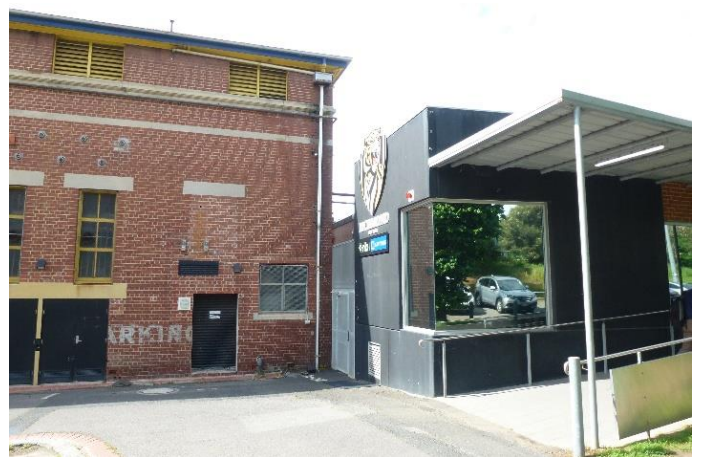
2022, Rear, join to administration building, new door and former window in brickwork
