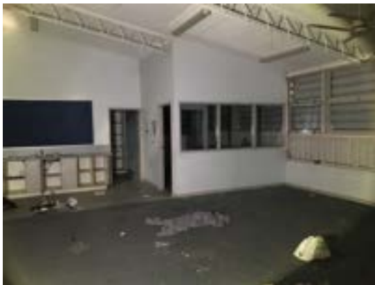
Classroom interior, representative of interiors throughout the 1880-1960s school building
