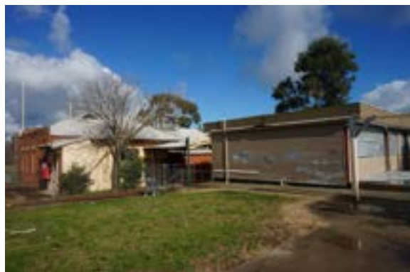
South of site, showing rear of fire station
