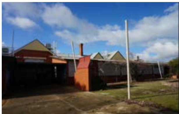
Western elevation of classrooms
