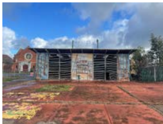
Shelter shed in the western portion of the school grounds
