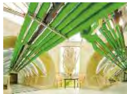
The distinctive pipe walkways at the former Clyde Cameron College. Images courtesy Murray Valley Private Hospital.
