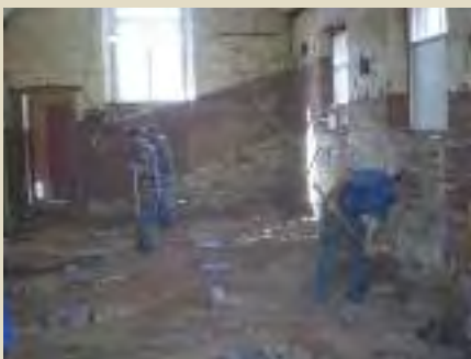
Below: Volunteers at work at Clydesdale Community Hall. The refurbished hall.
