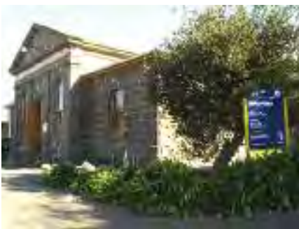
Extensive works are underway at the 1888 Portland Drill Hall, part-funded by $100,000 Heritage Grant, to replace flooring, external weatherboards, restoration of ceiling, internal truss roofing, etc. It had been in a very dilapidated condition.
