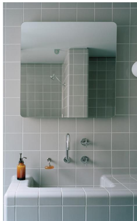
The kitchen and bathroom in the Kia Ora Apartment had been unsympathetically changed in a past renovation. These alterations were stripped out in a process of 'de-renovation'. The new facilities are clearly recognisable as new, while drawing on the aesthetic qualities of the Streamline Moderne apartment building.
