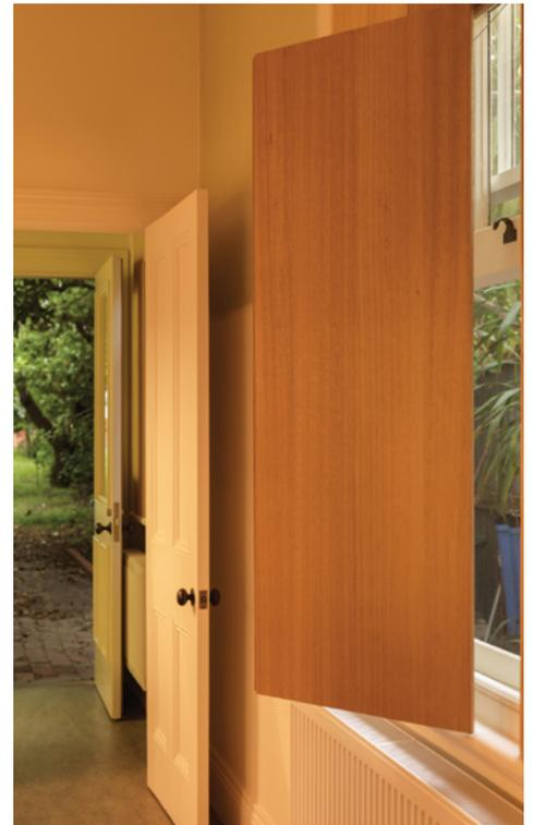
The Arnold Street House sought to retain as much of the original building fabric as possible. This is an inherently sustainable approach which retains embodied energy. Comfort and environmental performance was improved through the addition of delicately designed internal shutters, which improved thermal performance and meant the very thin original glazing could be retained.
