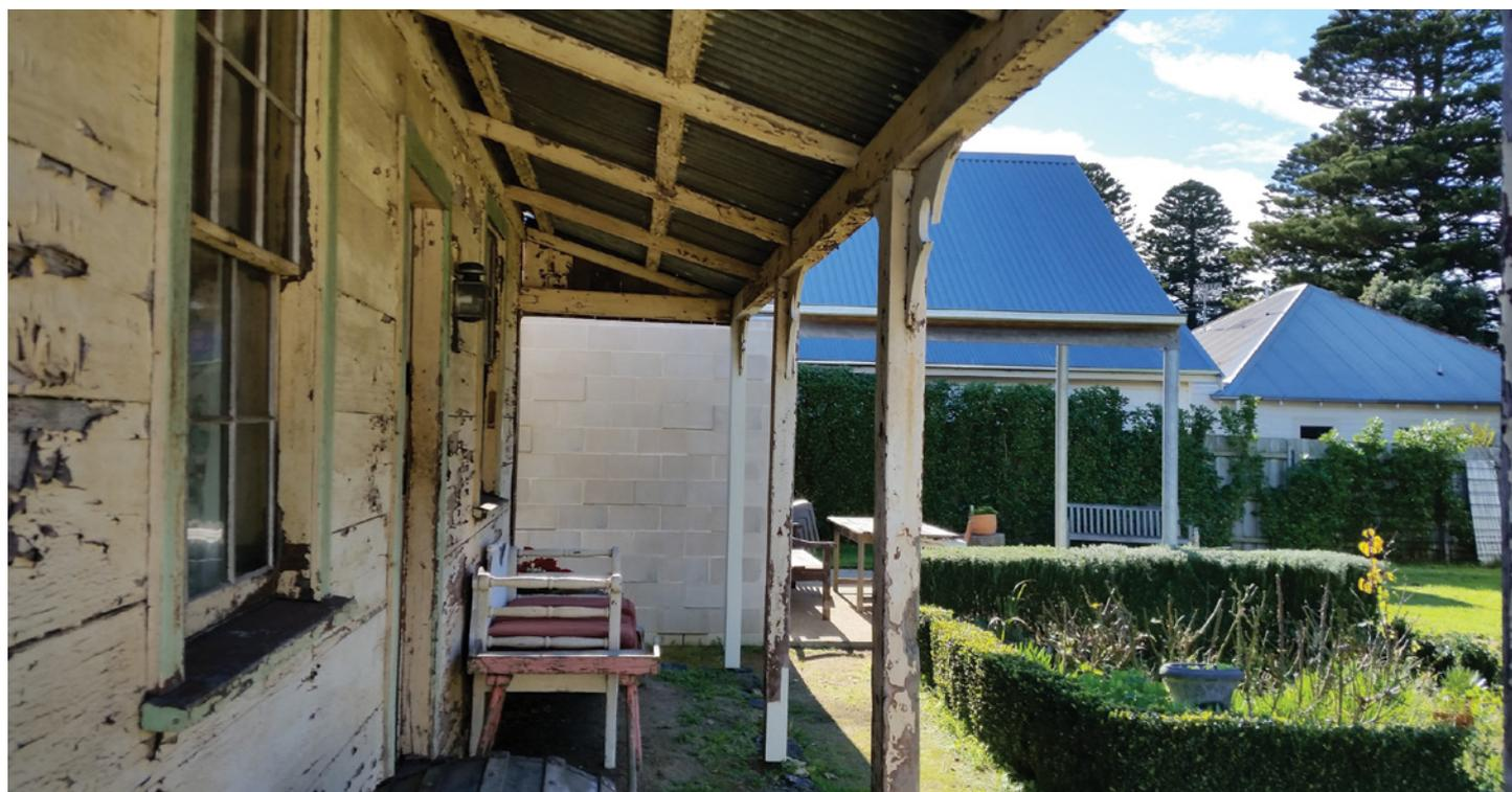
A very 'light touch' was taken at Kell Cottage, an 1840s house in Port Fairy. The structure was stabilised, exposed worn surfaces were patched and sealed, and the whole was cleaned. Finishes on surfaces that are protected from the weather were left as is, while new or exposed materials have been painted.
