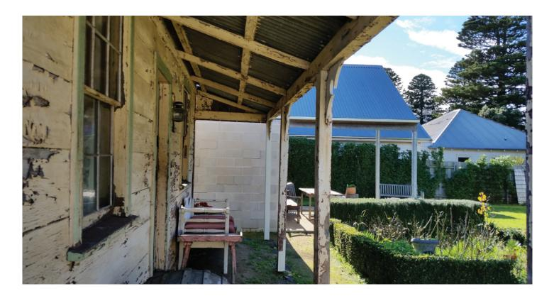
A very 'light touch' was taken at Kell Cottage, an 1840s house in Port Fairy. The structure was stabilised, exposed worn surfaces were patched and sealed, and the whole was cleaned. Finishes on surfaces that are protected from the weather were left as is, while new or exposed materials have been painted. ARCHITECT & PHOTOGRAPH: BRENDAN O'TOOLE ARCHITECT.
