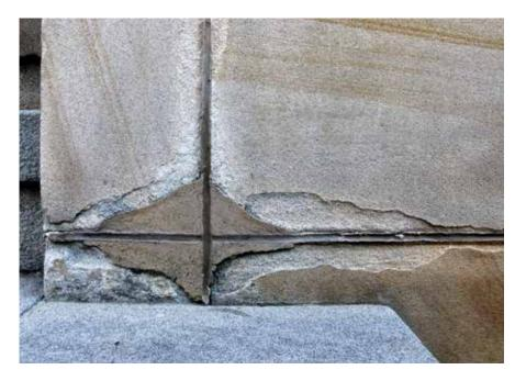
Penetration of water-repellent materials into the adjacent masonry can inhibit bonding of later repointing mortars.
