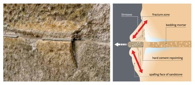
Figure 16: Spalling of edges due to thermal expansion.
