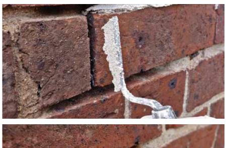
Figure 68: Filling a narrow perpend.
