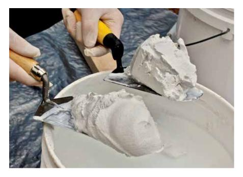
The densities of hydrated limes range from 350–640 g/L: that is, from about half to the same amount of lime per litre as in a dense putty. This has to be taken into account when batching: to make a mortar equivalent to a 1:3 mortar made with a dense putty may require a mix as rich as 1:2 hydrated lime to sand.
