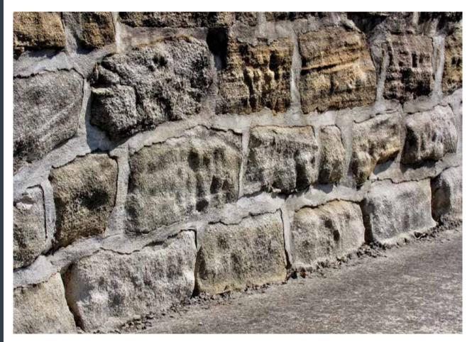
Figure 37: Incompatible mortar.
