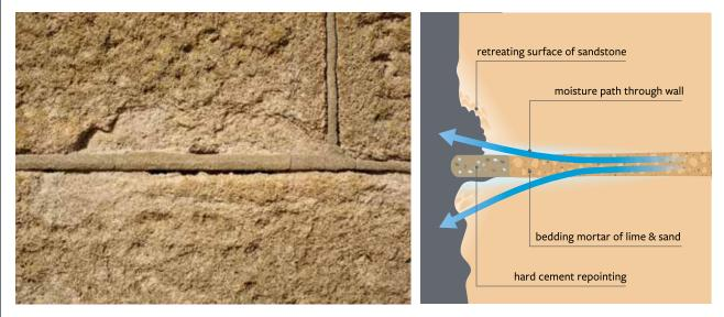
Figure 15: Impermeable mortar causing decay of adjacent stone.
