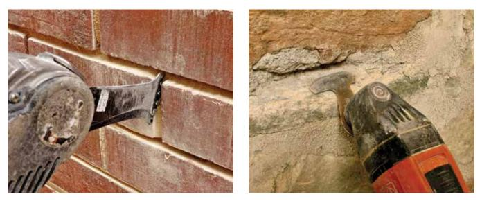
Figure 65: Oscillating-blade tools. These enable removal of moderately hard mortars while maintaining good control, reducing the risk of overruns. They are also much safer to use than rotating tools and produce less dust.
