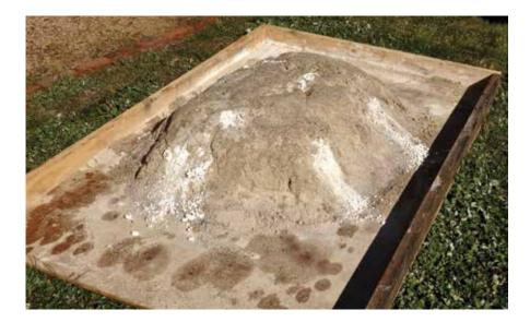
After cooling, the slakes were covered overnight to keep out any rain. The next day they were found to be still damp in parts, suggesting that the amount of water was about right for this particular quicklime and the dry sand. Less water should be added if the sand is damp. An advantage of this technique (unlike using lime putty) is that you can start with damp sand, as the quicklime will dry it (but you must allow for bulking).
