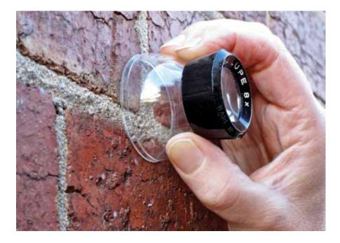
More powerful magnifiers in the range 15x–25x can be useful tools, particularly those that incorporate a scale bar as that enables measurement of sand grain sizes, while the magnification is sufficient to observe key features of the mortar. The benefits of magnifications higher than about 25x are offset by the unavoidably shallow depth of field – the distance between the nearest and furthest objects in focus.
