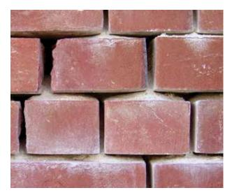
Figure 36: Compatible mortar.
