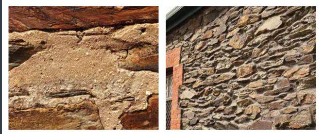
Figure 60: Flushed up pointing.
