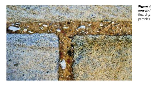
Figure 28: Shell fragments in an 1830s mortar. The rest of the aggregate is a very fine, silty sand with some darker gravel
