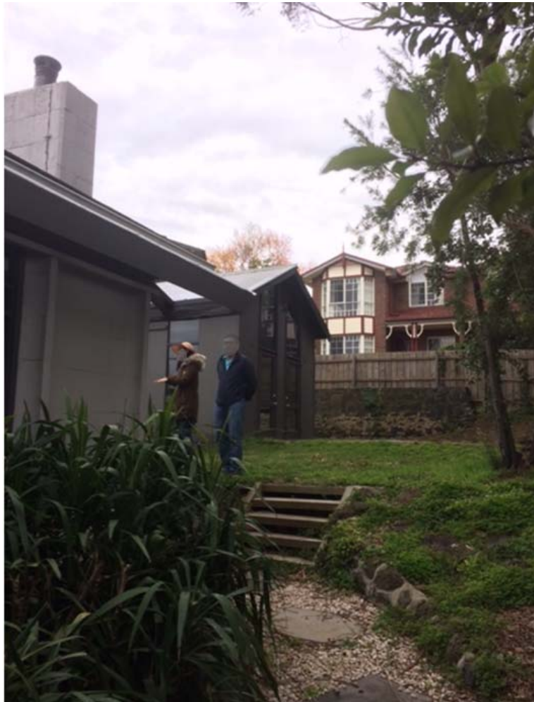
Northern elevation of the Jefferies House (front) showing the modern Dependent's Person Unit (DPU) (Rear). The 'barn' mentioned in the original extent is no longer extant.
