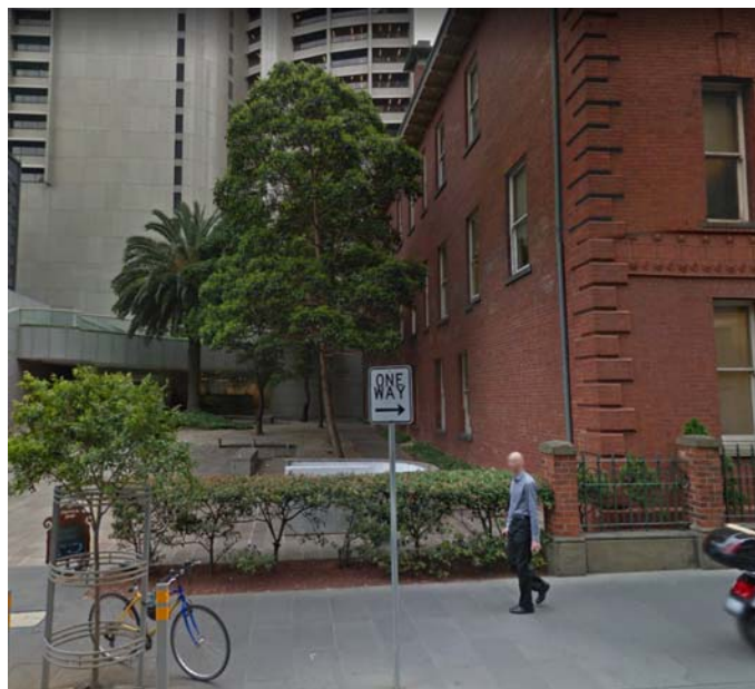
2017, View with No. 1 Spring on the left replacing the south wing.
