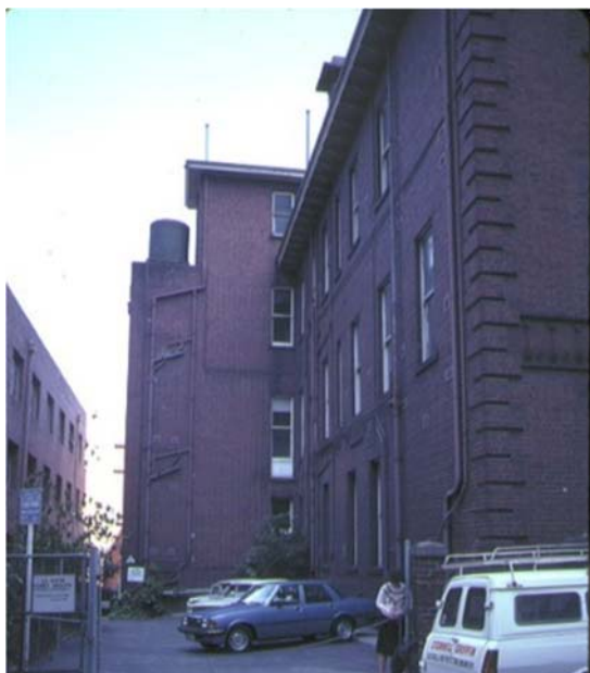
1982, View towards the south wing of Milton House.
