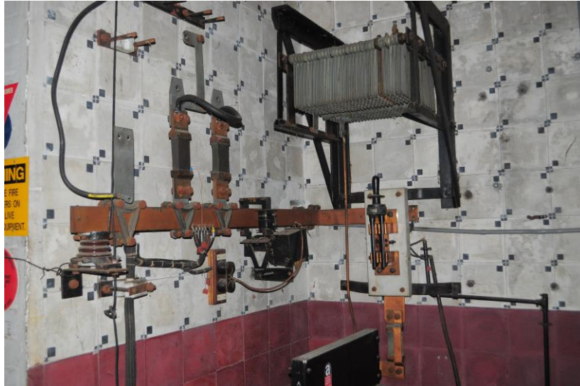
Interior of Deepdene substation showing tiles and rectifier equipment
