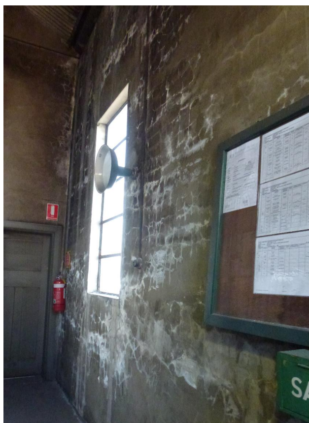
Interior showing salt efflorescence caused by damp, November 2019
