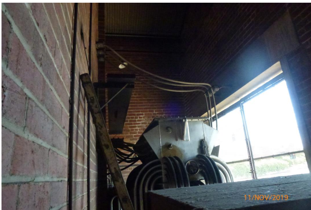
Top of transformer showing interconnected cables still present
