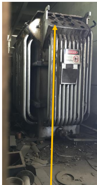
Transformer at Maribyrnong Tram Substation with cut cables at the top and vandalised components below
