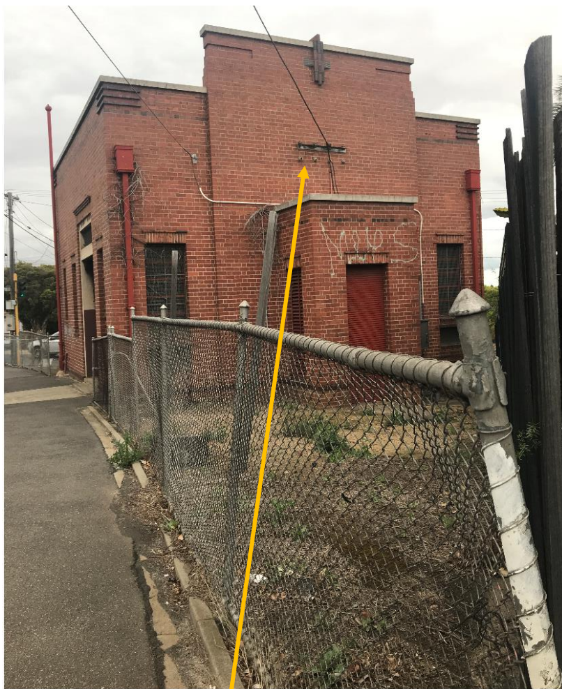
Rear of substation (north west) showing the bushes (holes where the positive DC cables exit the building to the tramlines) and the small room with roller door which houses the emergency resistance coils. November 2019
