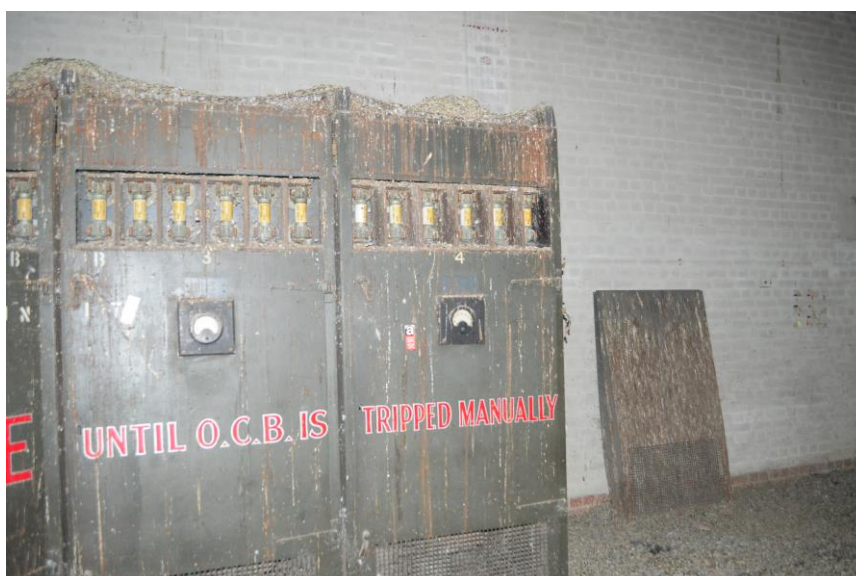
Essendon Tram Substation, empty rectifier cabinets and heavy deposit of bird droppings
