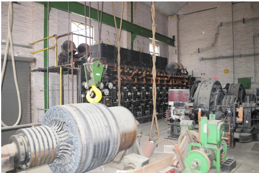
1929 Rotary converter rectification equipment at Malvern Tram Depot
