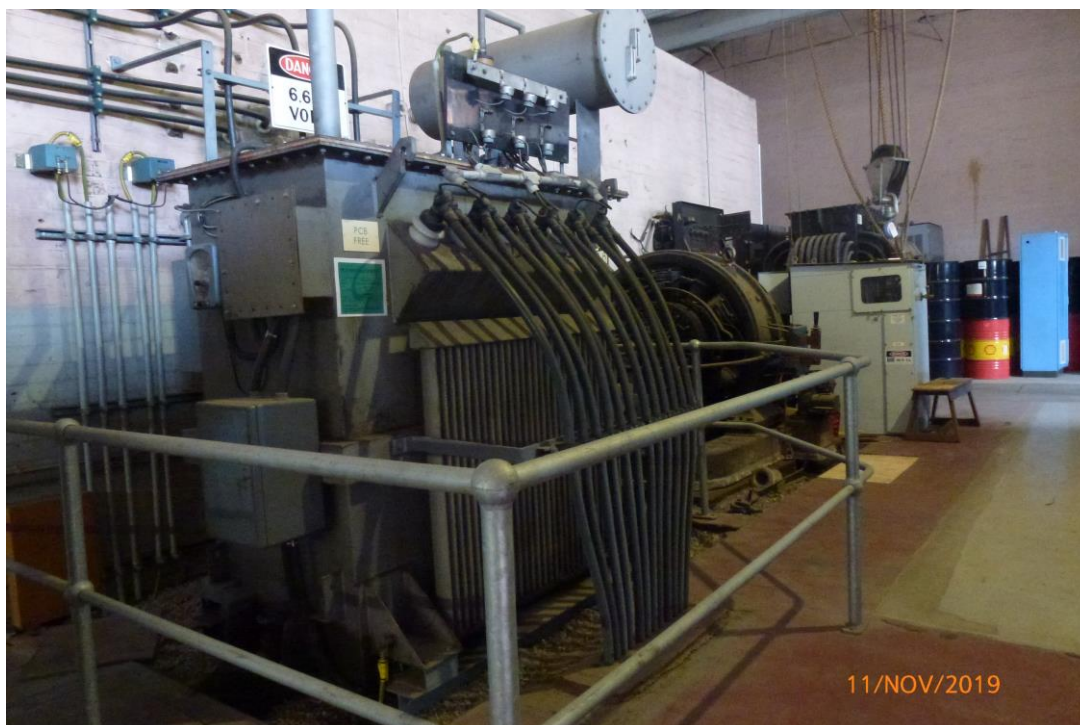
Transformer and rotary converter (not in original locations) at the former Cable Tram Engine House & Tram Substation, Brunswick
