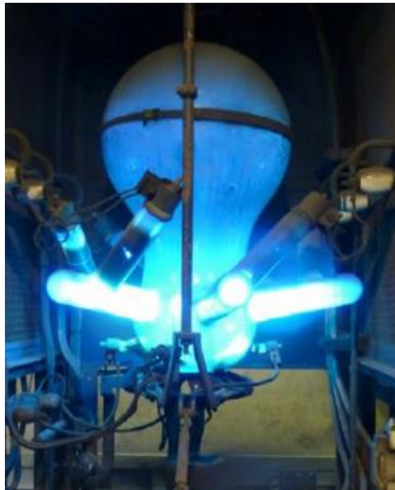
Glass bulb mercury arc rectifier in operation at Brunswick West Tramway Substation, March 2019. The eerie blue glow is vaporised mercury. Source: Nomination document.
