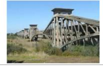
The **Ovoid Sewer Aqueduct** over Barwon River, Geelong (VHR H0895) is significant as an outstanding application of the Considere system of concrete reinforcement in a design derived from the steel Firth of Forth Bridge in Scotland. It enabled an overall length and span which exceeded any other reinforced concrete structure at the time of construction.
