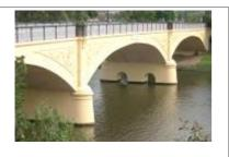
**Morell Bridge** over the Yarra River at Anderson Street, South Yarra (VHR H1440) is significant as the first reinforced concrete bridge built in Victoria (1899) – only two years after the first reinforced concrete bridge in the world - and the first in Victoria to use the innovative Monier construction technique patented by Joseph Monier, a French manufacturer of garden ware.
