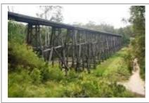
**Rail Bridge over Stony Creek**, Nowa Nowa (VHR H1436) is significant as a fine example of a timber trestle railway bridge, demonstrating the ingenuity and skill involved in constructing a railway line over a long distance, through difficult terrain and utilising local timber resources.
