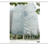
ICI House, Melbourne (VHR H0786) is significant for its considerable advancements in local construction techniques, including framed glazed curtain walls and innovative use of concrete, including precast reinforced units in structural members and flooring. The division of the glazed office space from the solidly clad service tower predates similar developments overseas.
