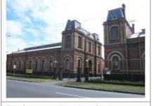
The **Sewerage Pumping Station**, Spotswood (VHR H1555) is significant as the key component of Melbourne's first centralised sewerage system which began operations in 1897. The station is unique in Australia as an intact ensemble of buildings, sewage pumping machinery and objects.
