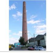
The **Shot Tower**, Clifton Hill (VHR H0709) is a rare as one of two surviving shot towers in Victoria. Its form reflects the shot production process: the shot was produced by dropping molten lead through sieves at the top of the tower into water at the bottom. The height of the tower allowed the shot to form before reaching the bottom.
