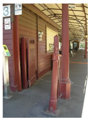
L: looking from the north along the edge of Platform 3 – the matching curvature of the canopy roof and platform edges is evident; R: painted cast iron and timber fence and gate components, beneath the northern end of the Platform 2 and 3 canopy. (Oct 2017)
