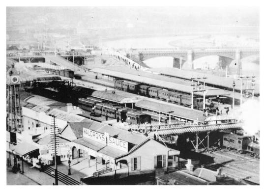
Flinders Street station (c.1887): the central of these three canopy platforms is the one that was dismantled and then reassembled in 1891 at Hawthorn Station's island Platform 2 and 3.
