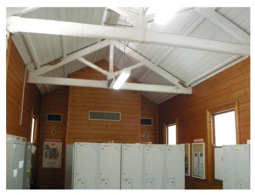
Looking north-east within the Burwood Rd end of the Platform 1 building. The king-post roof trusses abut those of the platform canopy outside the wall to the left. (Nov 2017)
