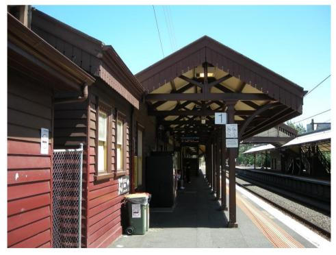
Looking southwards along Platform 1 at its buildings and canopy. The platform canopy's timber king-post trusses and support brackets of bent rail are visible. (Oct 2017)
