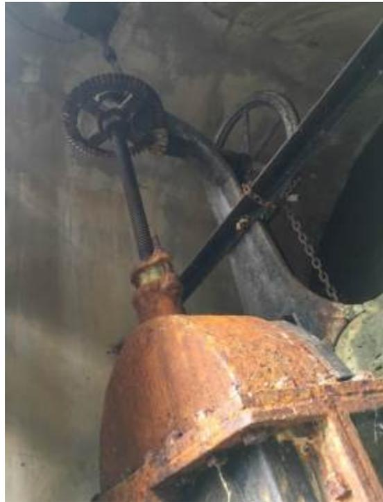
The water supply outlet valve in the eastern house. This took the water to the Anakie Gorge and joined the outlet pipes from Anakie Pipe Head Basin which pipes water to Geelong.
