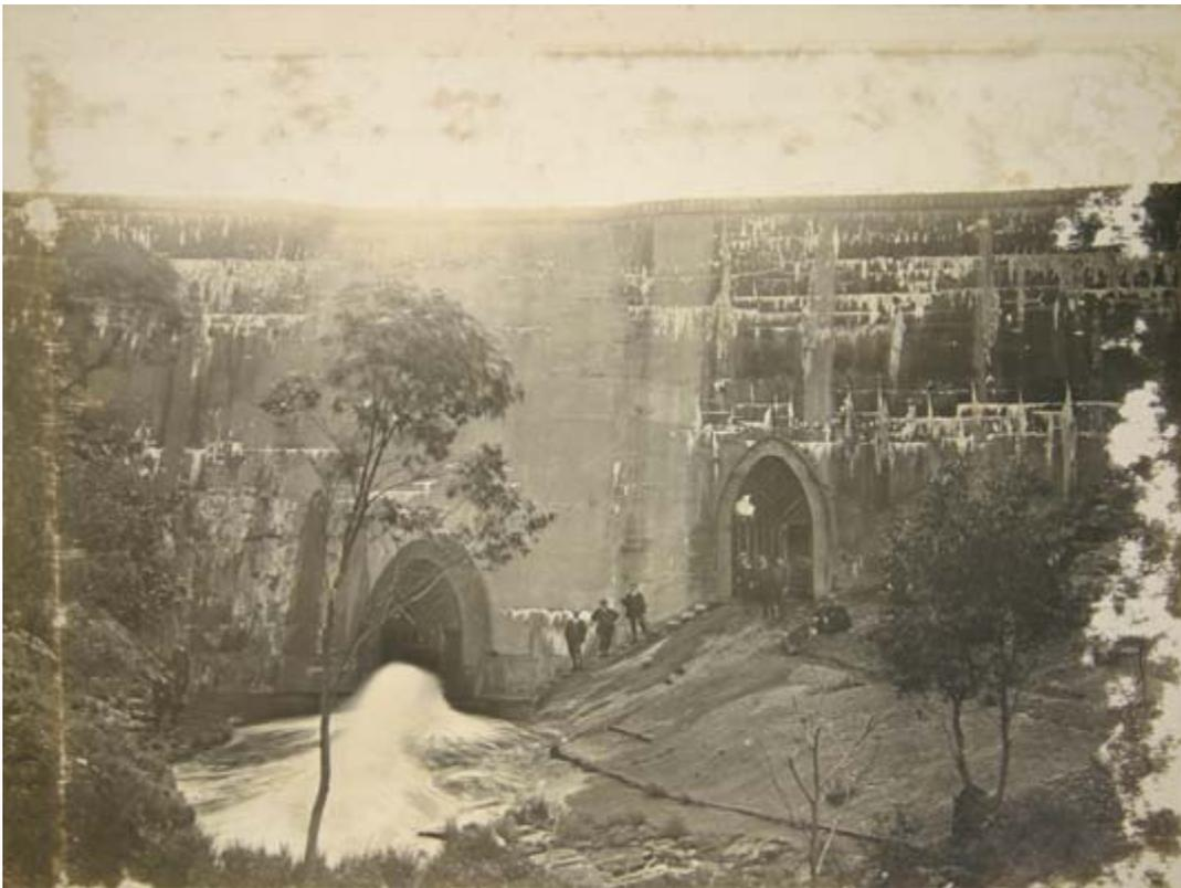
The outer face of the Lower Stony Creek Dam Wall c.1910 showing excess water being released from the outlet valve (Image: Geelong Heritage Service).
