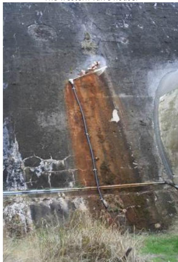
While the condition of the dam wall is good for its age, some cracks are being monitored. Proposed permit exemptions allow for such works to continue.
